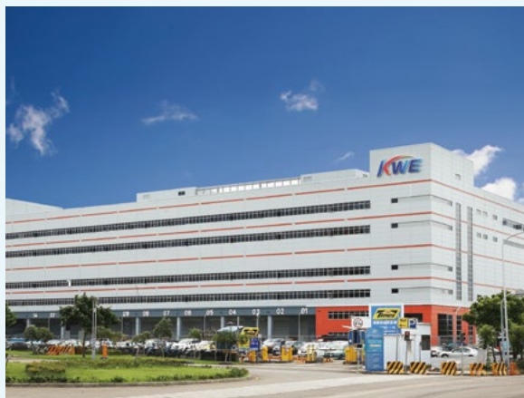
Taoyuan FTZ Terminal (Taiwan)
