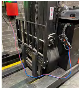
Electric forklift and charger
