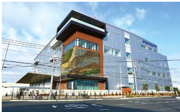
Misato Green Warehouse
