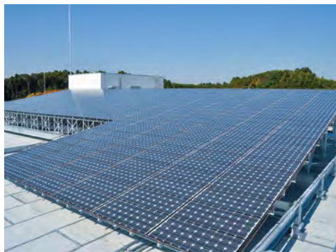
Narita Terminal solar power generating system
